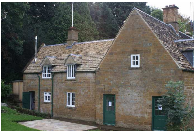
National Trust Cottage, Oxfordshire Domestic pellet boiler
