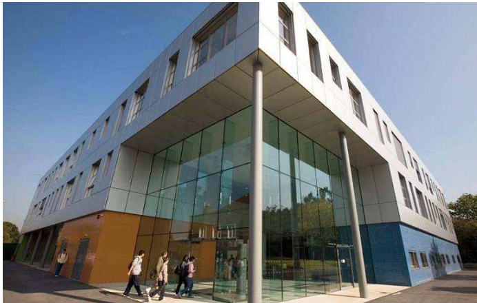
Chessington Community College wood pellet heating, Royal Borough of Kingston
