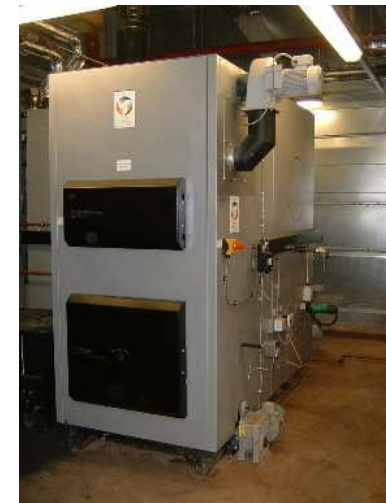
Hadley Learning Centre, Shropshire 320 KW wood chip boiler [PFI Project]
