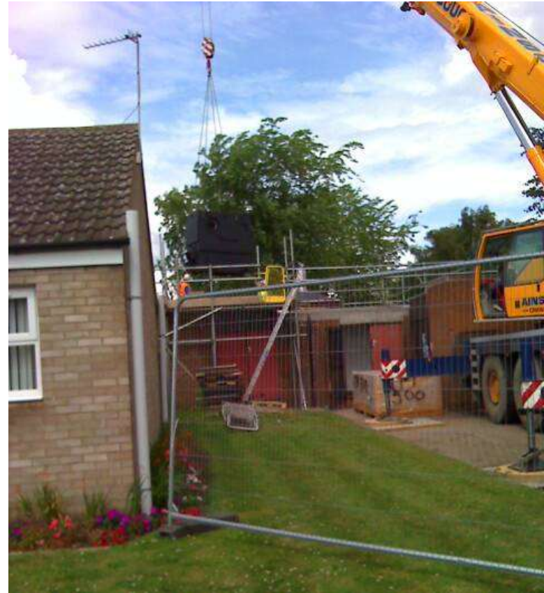
Froling 500KW boiler delivery into retrofit energy centre
