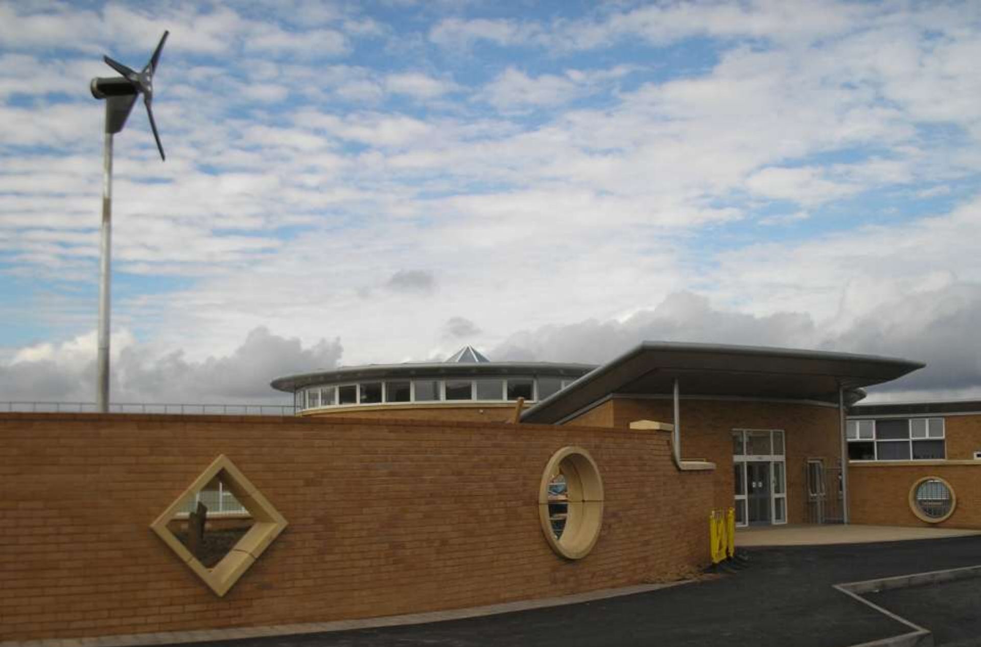
Fairfield Community Primary School
